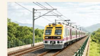
Central Railway Badlapur (Upcoming 3rd & 4th Line)
